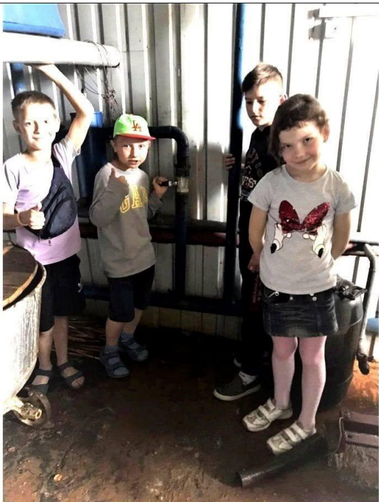
SOME OF THE ORPHANS ARE CHECKING OUT THE NEW WATER SYSTEM & PLUMBING WE FUNDED & HAD INSTALLED AT THEIR ORPHANAGE. I LOVE THIS PICTURE THEY SENT
