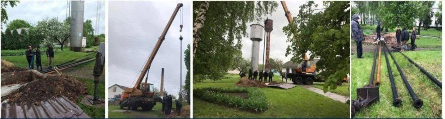
NEW WELL, PIPING, WATER PUMP, AND INSIDE PLUMBING WE FUNDED AT KOMARIVKA ORPHANAGE
